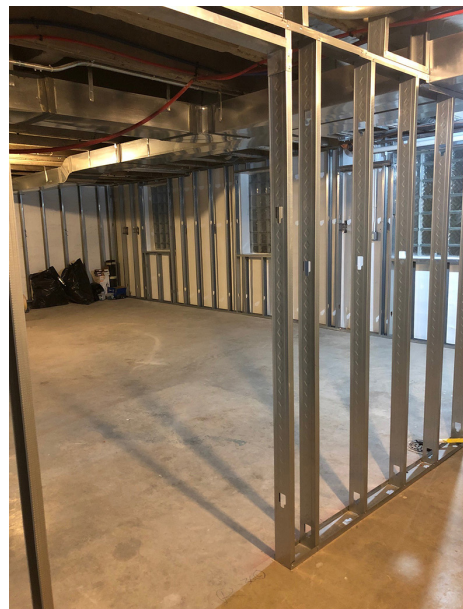
The renovated basement will include a new classroom, restroom, workshop, storage areas and an open sitting area. Pictured above is framing for the new classroom.
